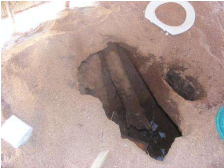
*The toilet after the initial collapse – despite being repaired with concrete, it somehow still managed to act as a near-death-trap!*
